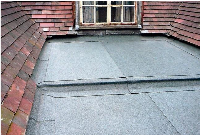
Pitched roof abutments
