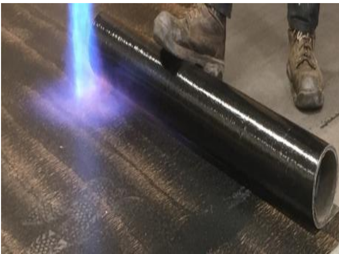
Figure 3 - Typical torch on method of application
