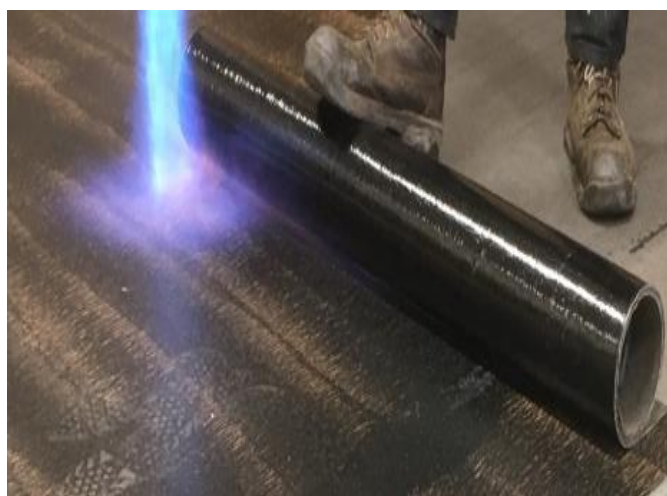
Figure 3 - Typical torch on method of application
